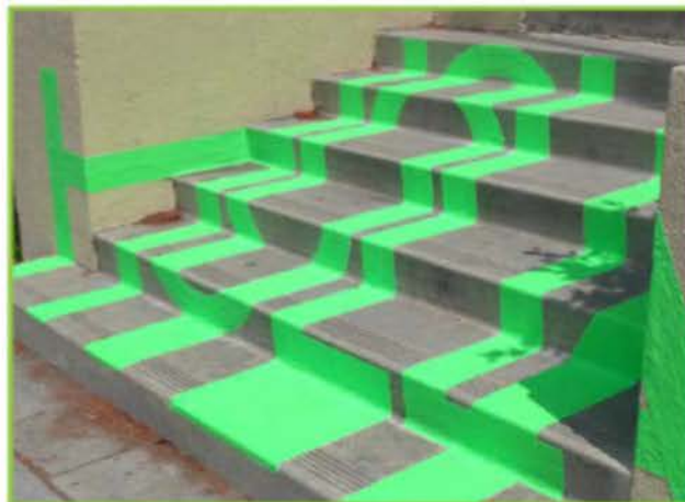
Historic Civic Center, detail
