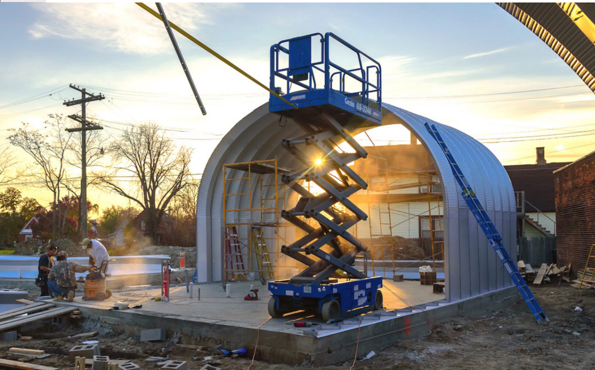
Image: Construction of True North in Detroit, Michigan
